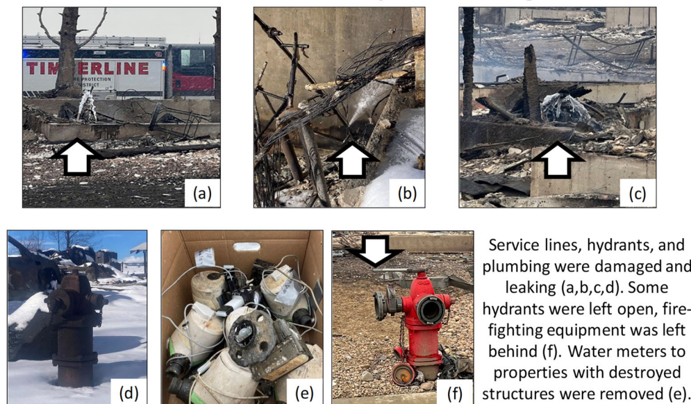
FIGURE 2 Water systems experienced different degrees of damage as service lines, hydrants, and property plumbing were damaged and leaking, and source water and treatment and facilities were also impacted.
